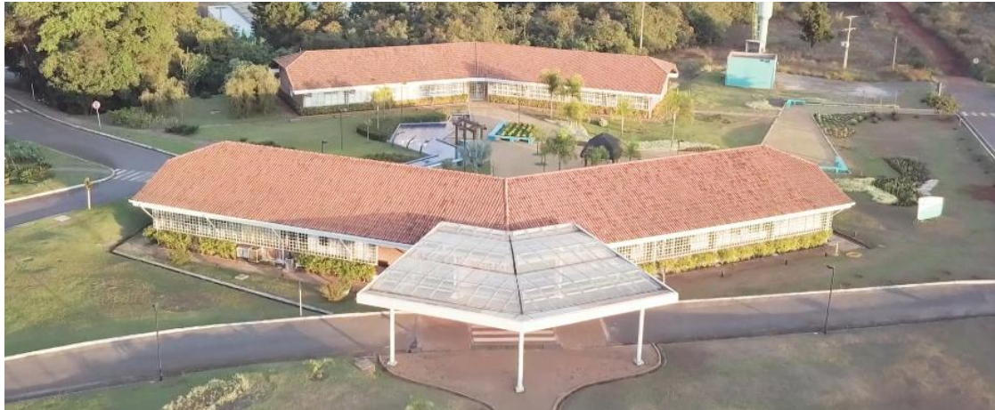
Vale's Ferrous Technology Center (CTF) in Nova Lima, Minas Gerais, Brazil
