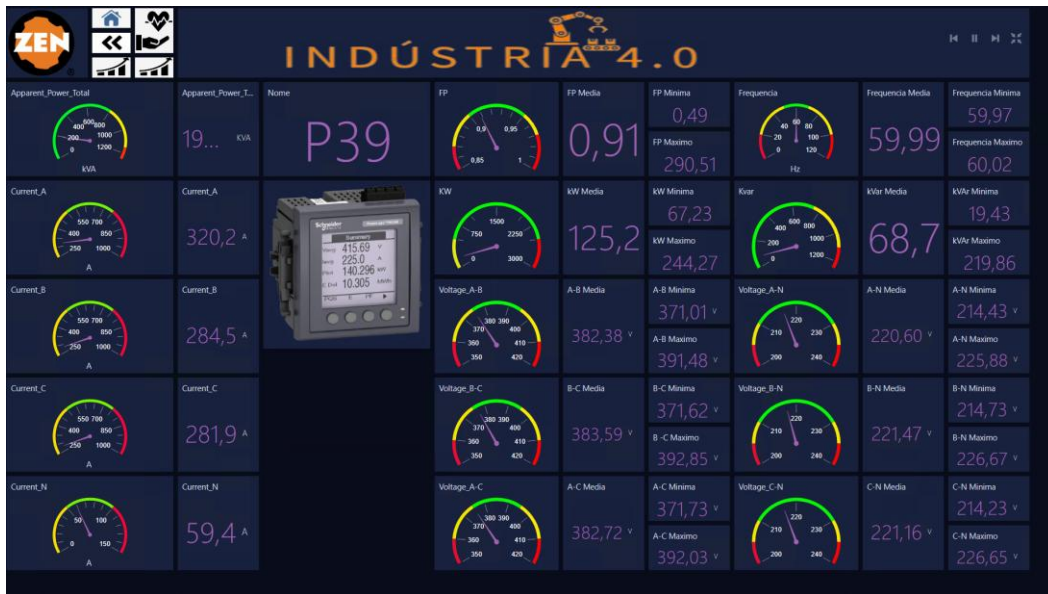
Controlling measured variables from a power multimeter
