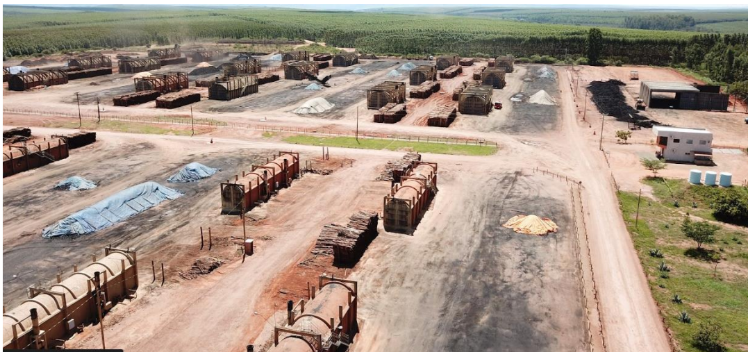
Carbonization kilns at Palmeiras REP
