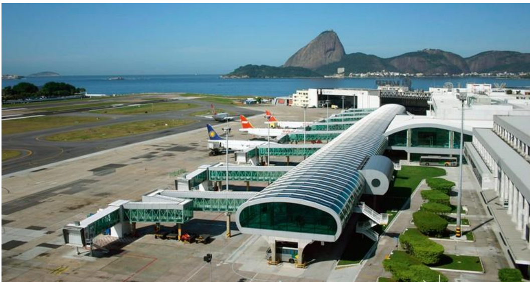
A single operations center at Santos Dumont Airport can control the three airports
