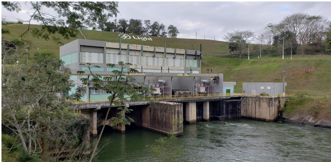
Santa Branca hydro power plant
