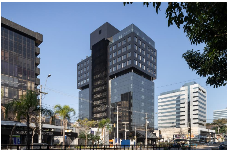
Figure 1. JBZ Building, the most sustainable in its category in south of Brazil
