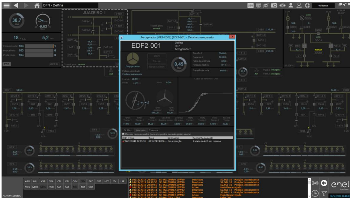
Controlling a turbine at Delfina wind farm
