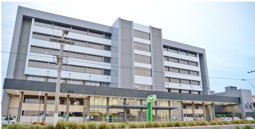
Figure 1. Unimed VTRP facility in Lajeado, RS
