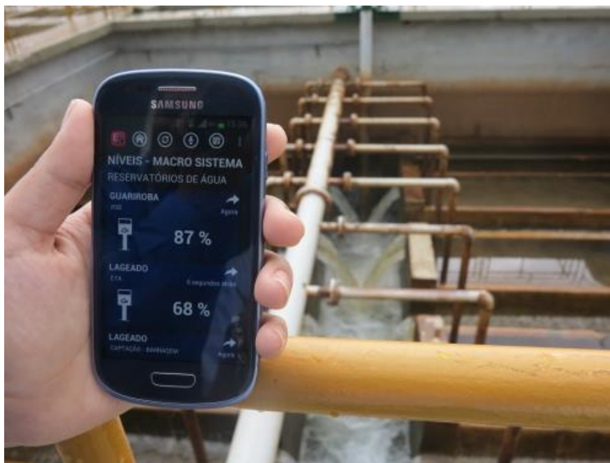
Figure 1. A controller monitors the reservoirs' water level via Elipse Mobile from a smartphone
