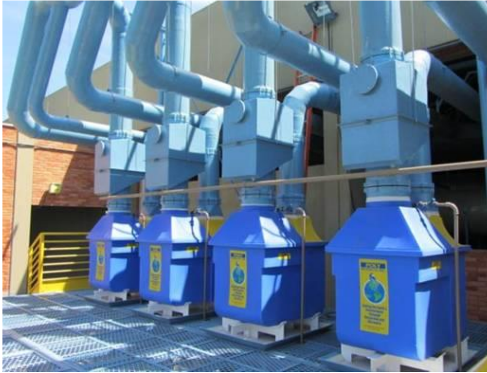
Figure 9. Hoods used for treating air from the plating process before releasing it to the atmosphere
