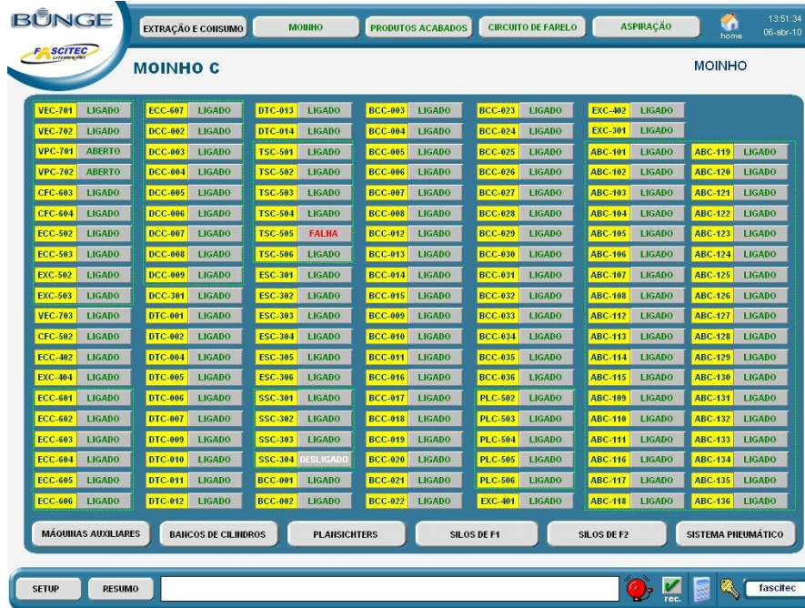
Figure 3. General view of the equipments
