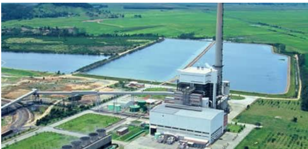
Figure 1. Jorge Lacerda Plant C
