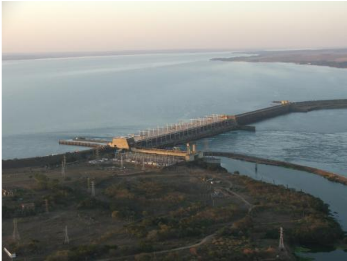
Figure 3. Engenheiro Souza Dias (Jupiá) hydroelectric plant
