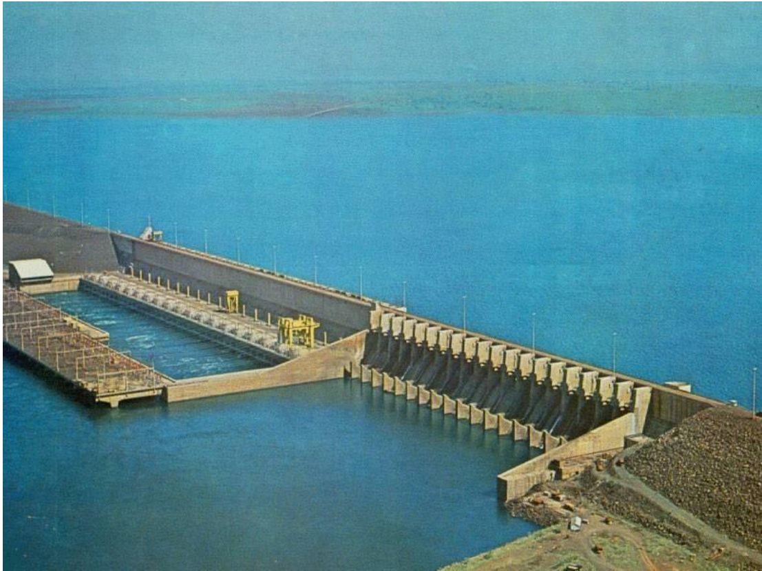
Figure 2. Ilha Solteira hydroelectric plant
